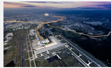
Brisbane Airport Expansion | $2.4 Billion
