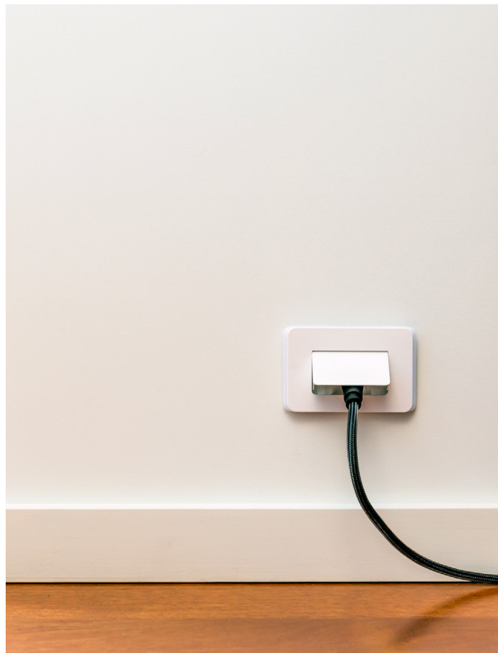
Aesthetically appealing cable management
