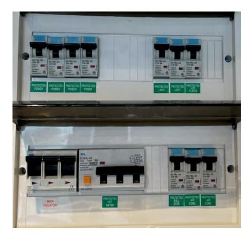
In addition to your Mains switch, there are safety switches/circuit breakers for the apartment power points, light fittings, wall oven, hot water system, and air conditioning unit.
