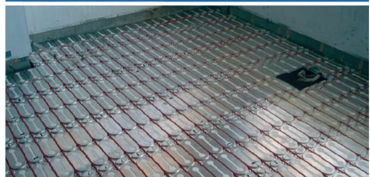
Insulated Heating Panels for Under Floating Floors
