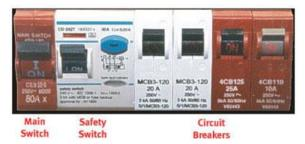
**Typical switchboard** – this shows the main switch, safety switch with test button, and four circuit breakers. All homes have circuit breakers or fuses. These are designed to protect the wiring and appliances within the premises. Only safety switches are designed to protect people.
